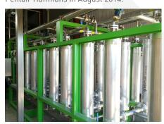
In order to inject gas into the grid, it has to meet certain specifications', explains Pentair Haffmans sales manager Mr. Francois Huberts. 'Biogas consists of roughly 55 percent methane and 45 percent carbon dioxide. It turned out that the supplier of the digester could not deliver a system that included  $\mathrm{CO}_2$  recovery. In fact, some of the methane would also be lost with their Pressure Swing Adsorption or PSA process.
