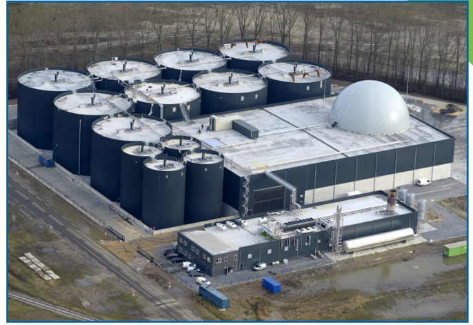
Aerial view of the Biogas Upgrading Plant of SFP Group in Westdorpe, NL
